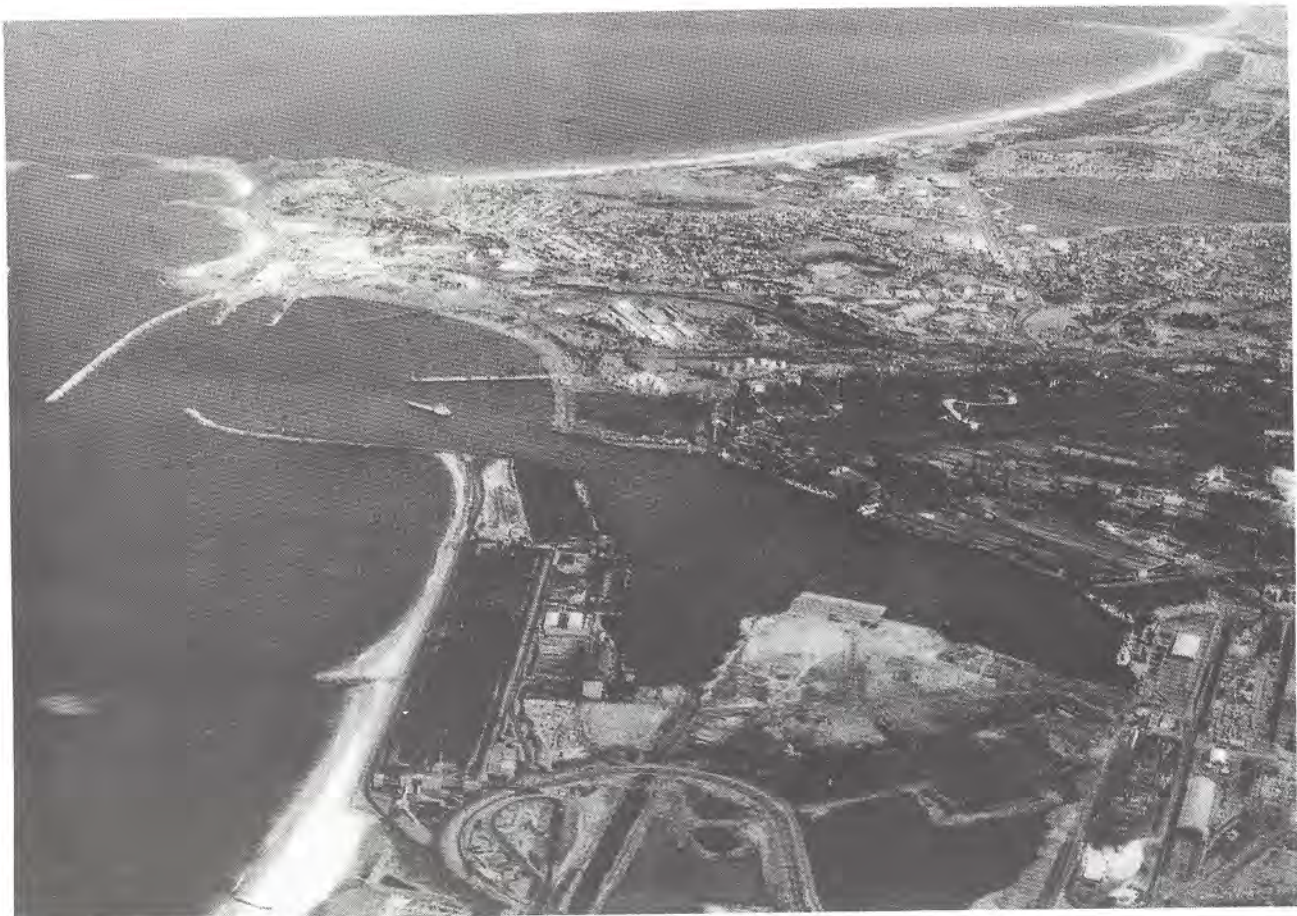
Fig 1.33: A Port has to be specially constructed to avoid the refraction patterns of waves. Photo courtesy of NSW Maritime Services Division - Port Kembla
