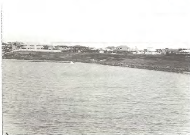
Fig 3.44. Then build houses on the dredged out sand.
