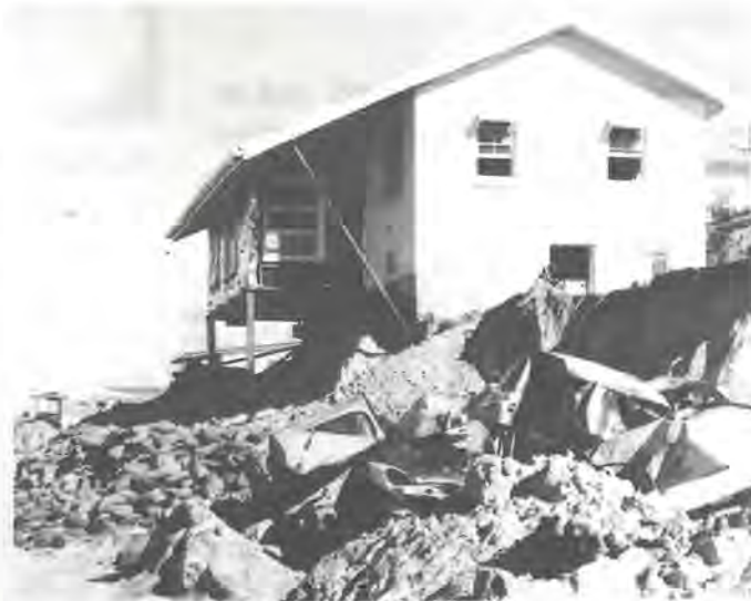
Fig 3.8: Beach erosion can cause problems. Photograph courtesy Beach Protection Authority
