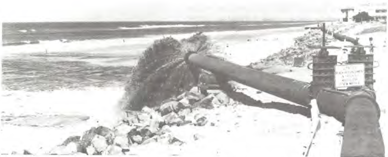
Fig 3.23 Beach nourishment involves adding sand to the sand budget from outside the active beach system. Here sand is pumped from a river to the beach as is illustrated by method 3 below. Photograph courtesy Beach Protection Authority.
