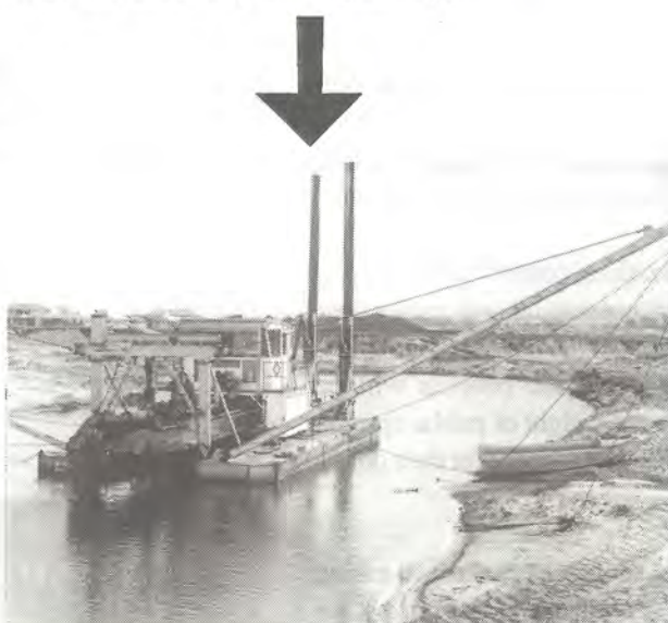
Fig 3.43. Dredge out the sand to make a canal and pump it up into a walled off area
