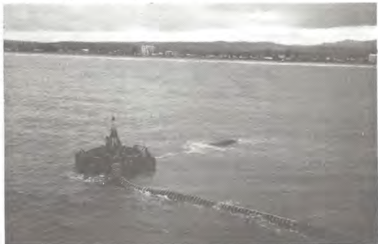
Fig 3. 27: Once the dredge had finished sucking up the sand, it moored at a pontoon where the sand from the hopper is pumped ashore.
