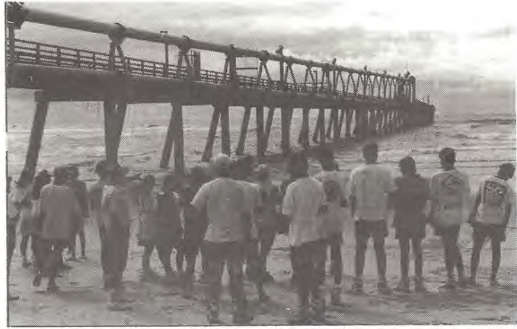
Fig 3.36: The sand pumping jetty at the new seaway entrance.
