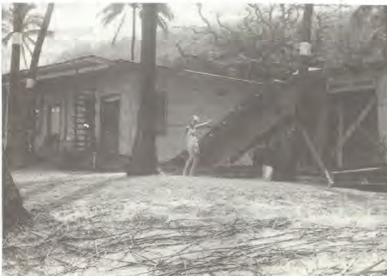
Fig 1.19: This house was demolished by a huge wave run-up on Hawaii's North Shore.
