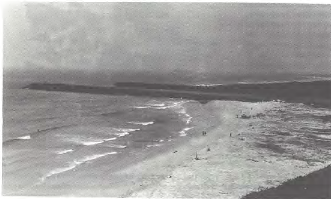
Fig 3.6: Training walls result in sand being trapped for a time behind the wall on the side of the prevailing winds
